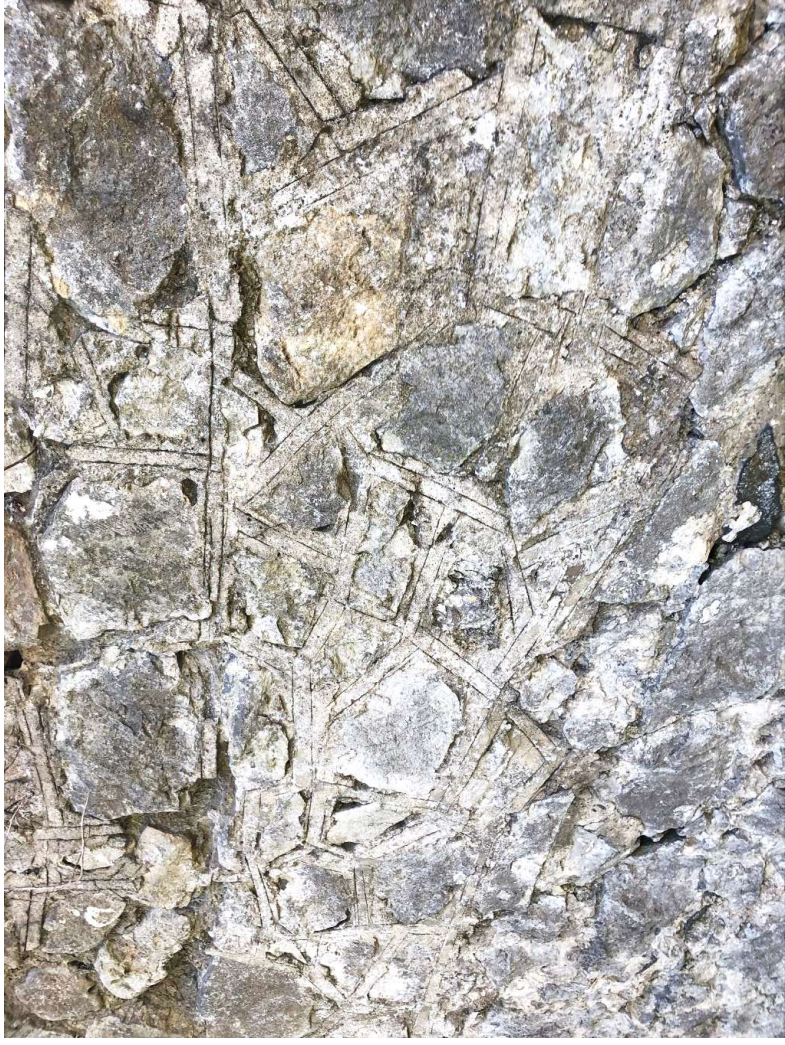
52. Detail view of the boundary wall to the northern boundary of the subject site
