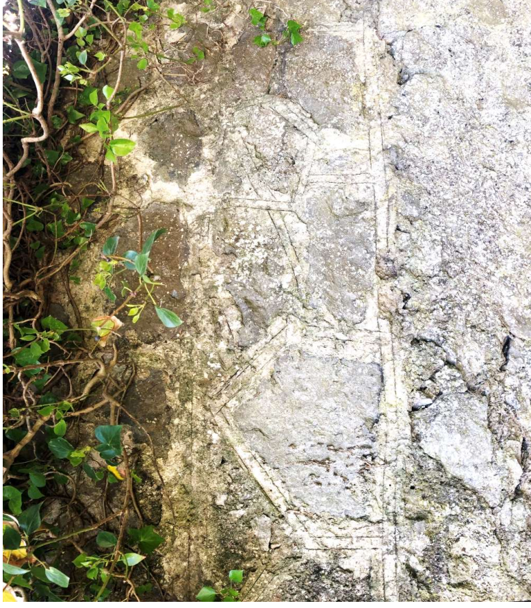
10. Detail view of the historic demesne wall to Howth Castle
