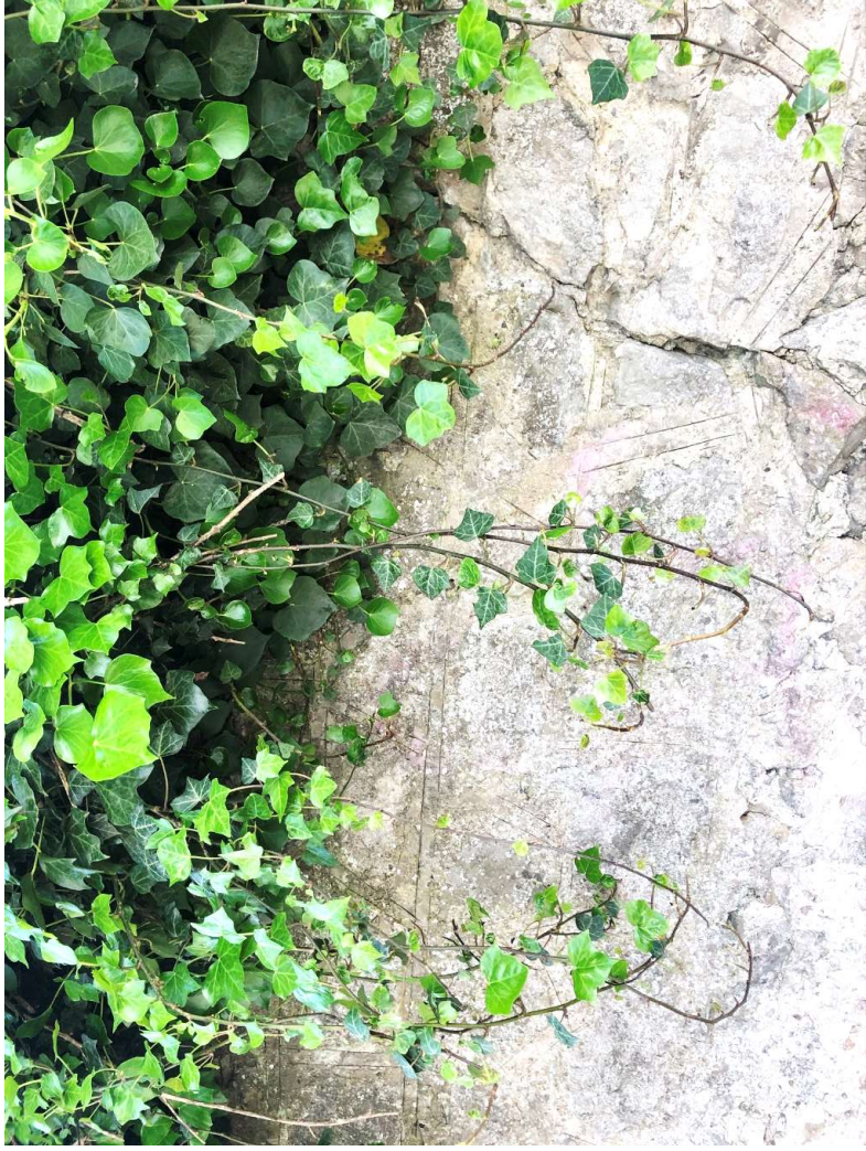
50. Detail view of the boundary wall to the northern boundary of the subject site
