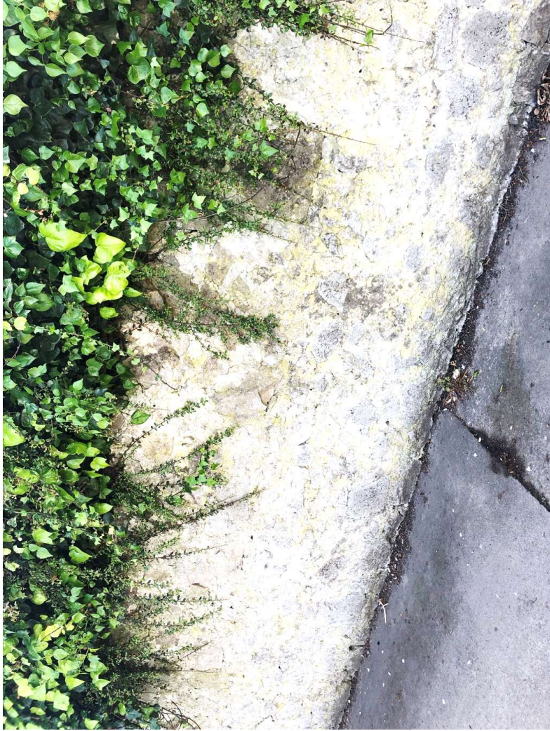
43. View of the historic demesne wall to the west along Howth Road
