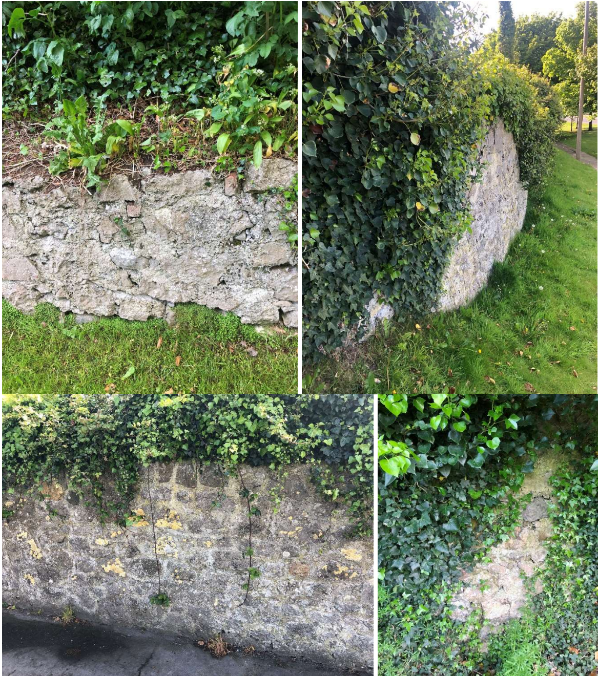
Figure 4: Photographs along the historic boundary wall to the northern and eastern boundaries of the subject site
